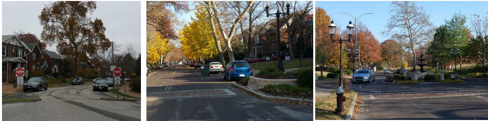
Examples of traffic calming techniques in neighborhoods (from left): an exit-only street connection between a neighborhood and a major street; bulb-outs (which also create a shorter pedestrian crossing); and a traffic circle.
