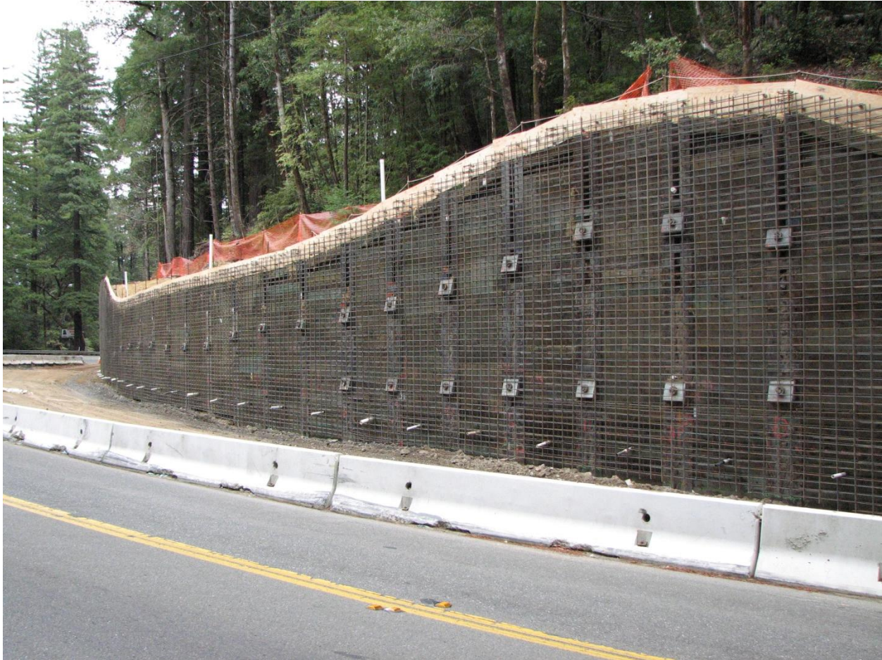
Tieback Wall before shotcrete facing
