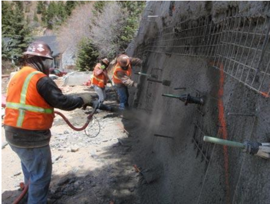
Soil Nail Wall Construction
