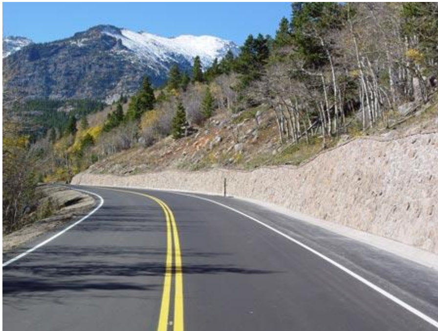
Completed Soil Nail Wall
