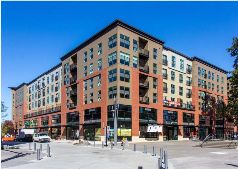
Figure 12. The Rowlock at the Platform District at Orenco Station
