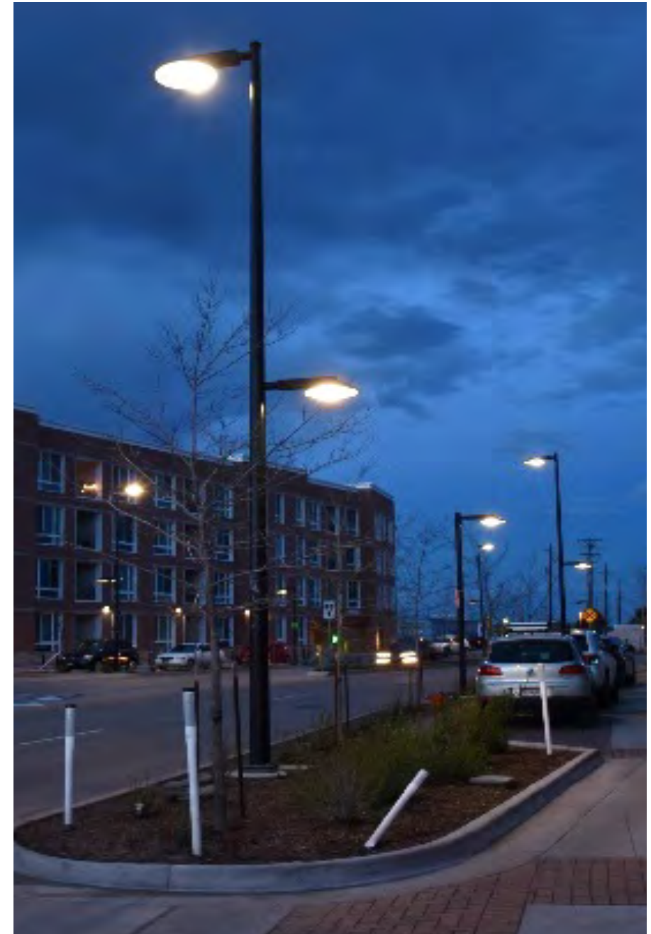
Lights with low glare provide more comfortable streets and public spaces, providing light where it is needed without annoying nearby residents. Source: (SLC Street Lighting Master Plan)
