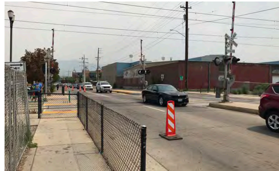
Current north access to the Ballpark TRAX Station / GSBS Consulting
