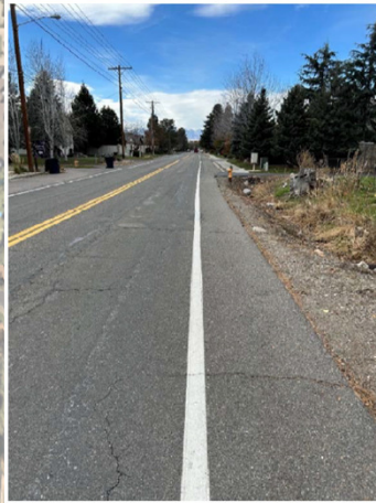
6400 South at 1765 East: Looking West
