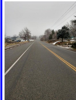
Figure 5: SR – 106 (200 East) Existing Conditions
