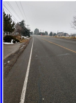
Figure 2: SR – 106 (200 East) Existing Conditions
