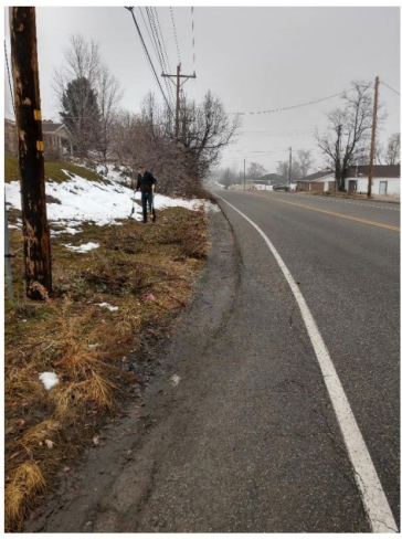
Figure 3: SR – 106 (200 East) Existing Conditions
