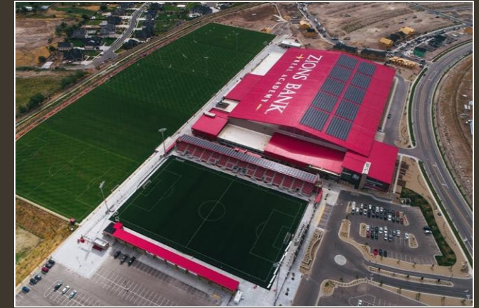
Zions Bank Soccer Stadium
