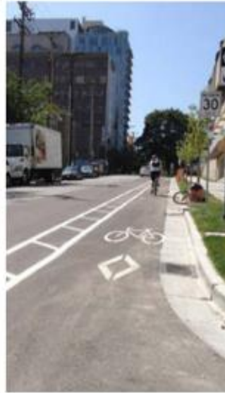
Paint Buffered Bike Lane
