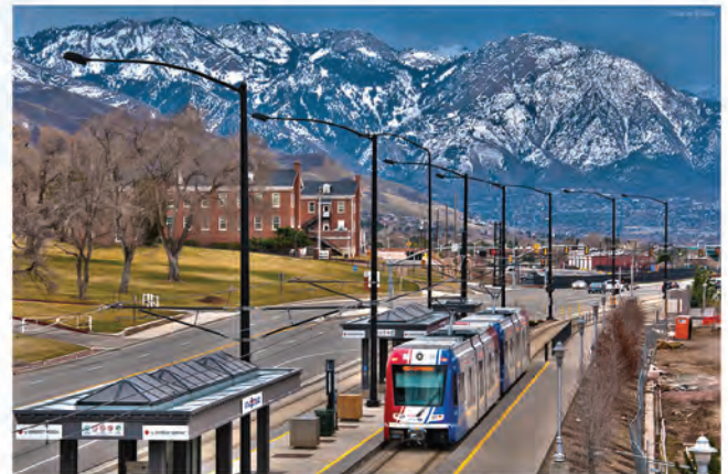
FTA grants supported construction, operation of Utah Transit Authority's TRAX light rail.
