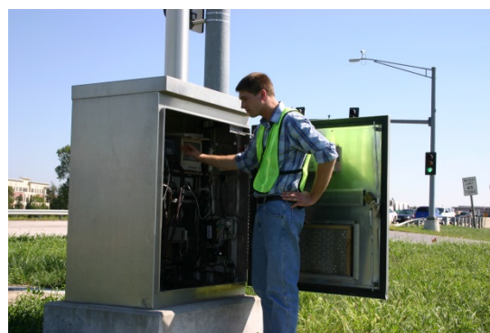
Figure 19 Operation Green Light technician adjusts signal timing at traffic signal cabinet. Source: MARC
